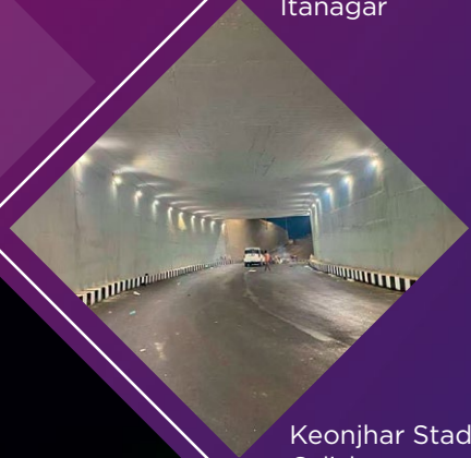
Tunnel lighting, Itanagar
